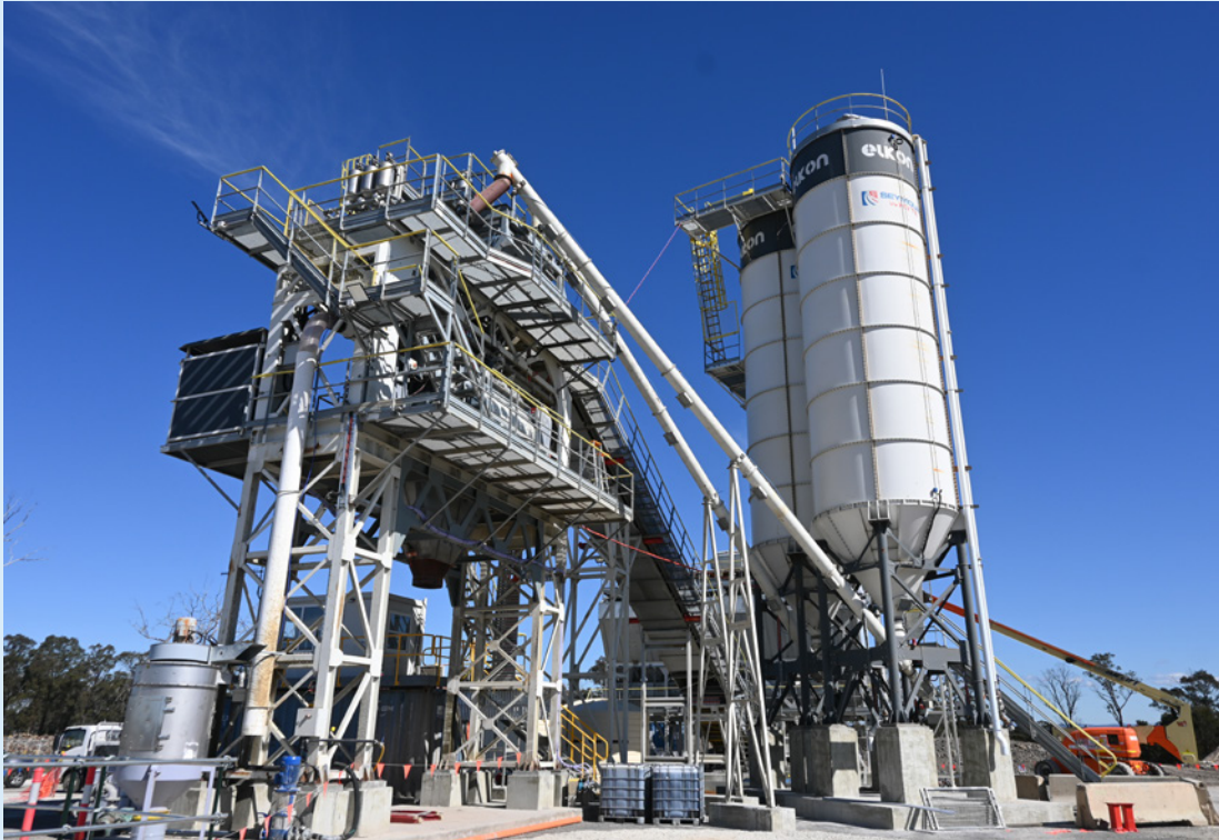
Concrete batch plant on Clifton Avenue Kemp's Creek
