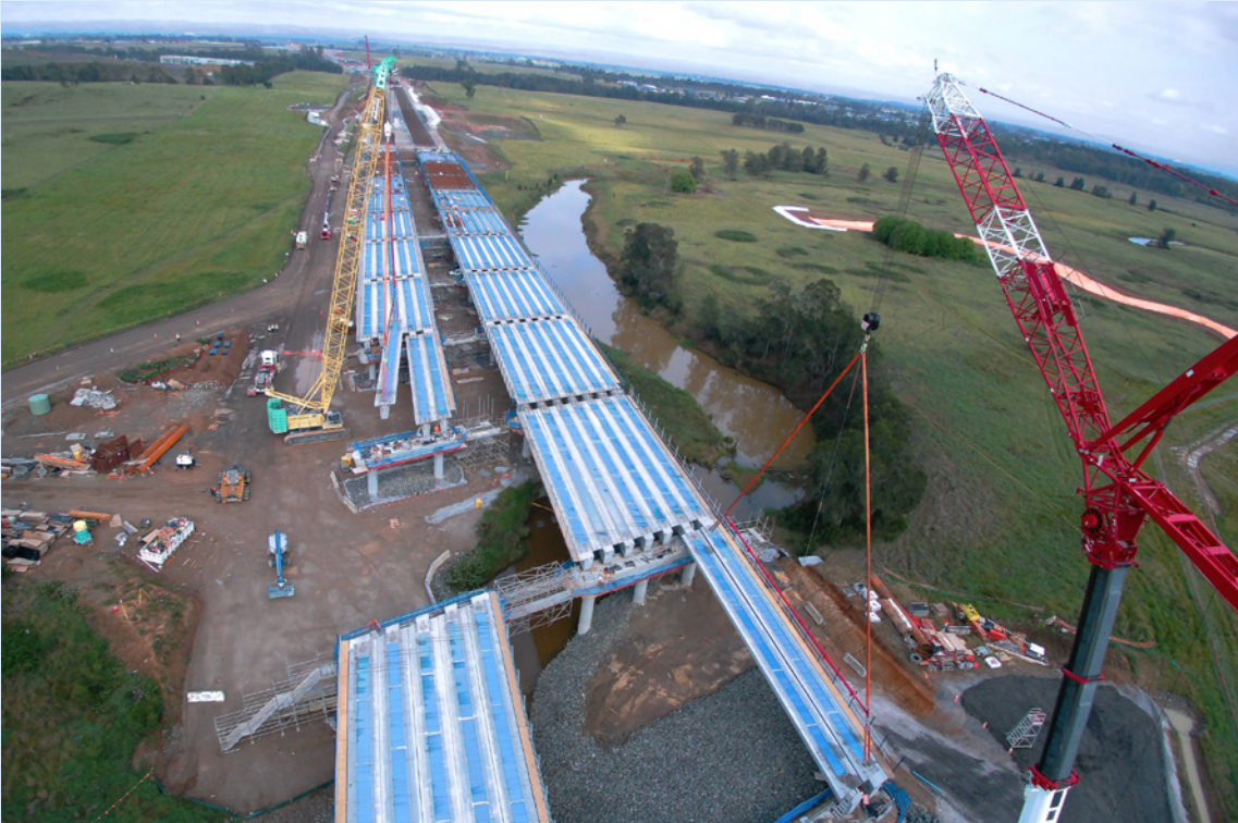
South Creek bridge girder installation
