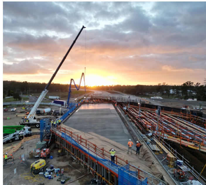
Elizabeth Drive bridge near Mamre Road in Kemps Creek
