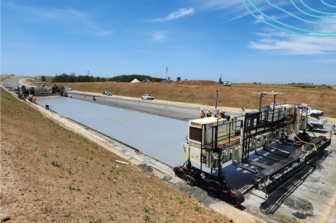
First mainline pavement trial at The Northern Road
