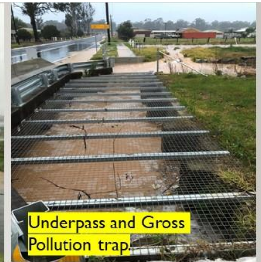
Underpass drains blocked causing road flooding.
