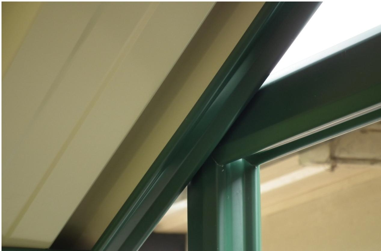
Vertical posts attach to "A" frame next to horizontal bracing. Photo shows two posts interlocked and screwed together for additional strength. Same applies to the horizontal bracing, without the interlocking rail a "channel only" post or bracing would look less attractive and have far less strength, especially for those keen on "chin-ups" .
