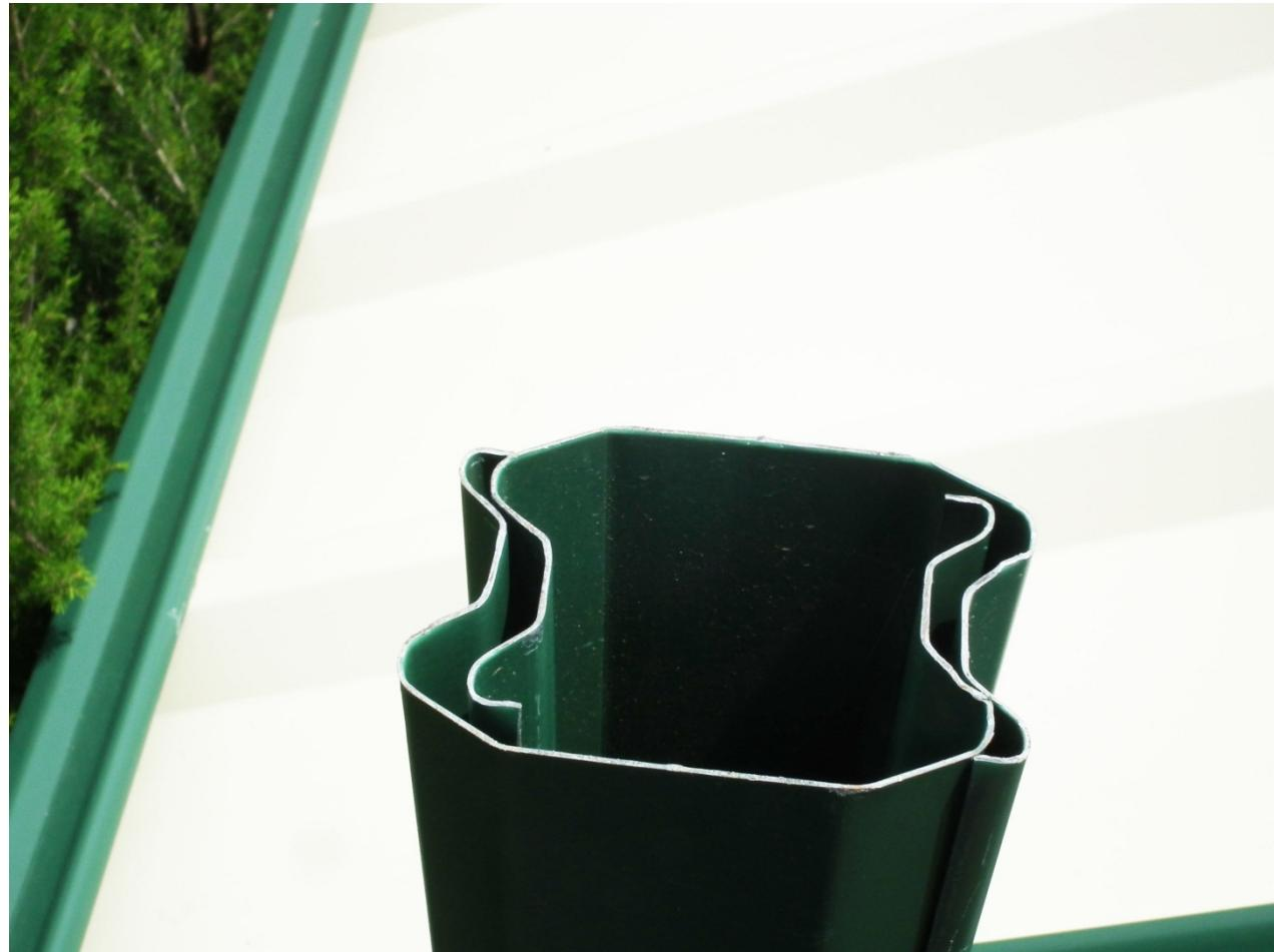
Galvanised self threading screws pull the sides of the posts together to form a single post. This was done to the 4 vertical posts and the two horizontal bracing “rails” which are actually fence posts. I used 6 screws per post, 2 each end and 2 in the middle. To make it easier, predrill holes for the self threading screws. First a small hole through both walls, then a clearance hole in the outer wall only. This is where two drills and socket driver are very handy.
