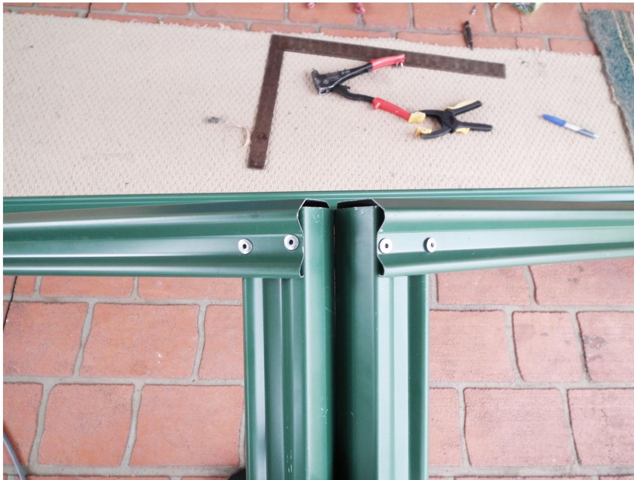
That's where it's going – using the existing fence posts. Distances are crucial, measure carefully for the next step. 2 BBQ Pergola posts are pop riveted to the existing fence posts. Another 2 posts are pop riveted to the "A" frames, these then fit inside the posts previously riveted to the fence posts! A few mm out and it wont fit! So measure several times, make sure you know what fits where!
