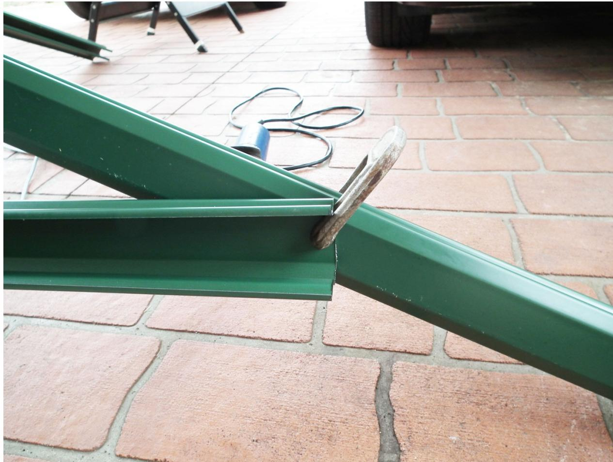
One half of Roof – A frame. 2 sheets per side then locked in place by bottom rail.
