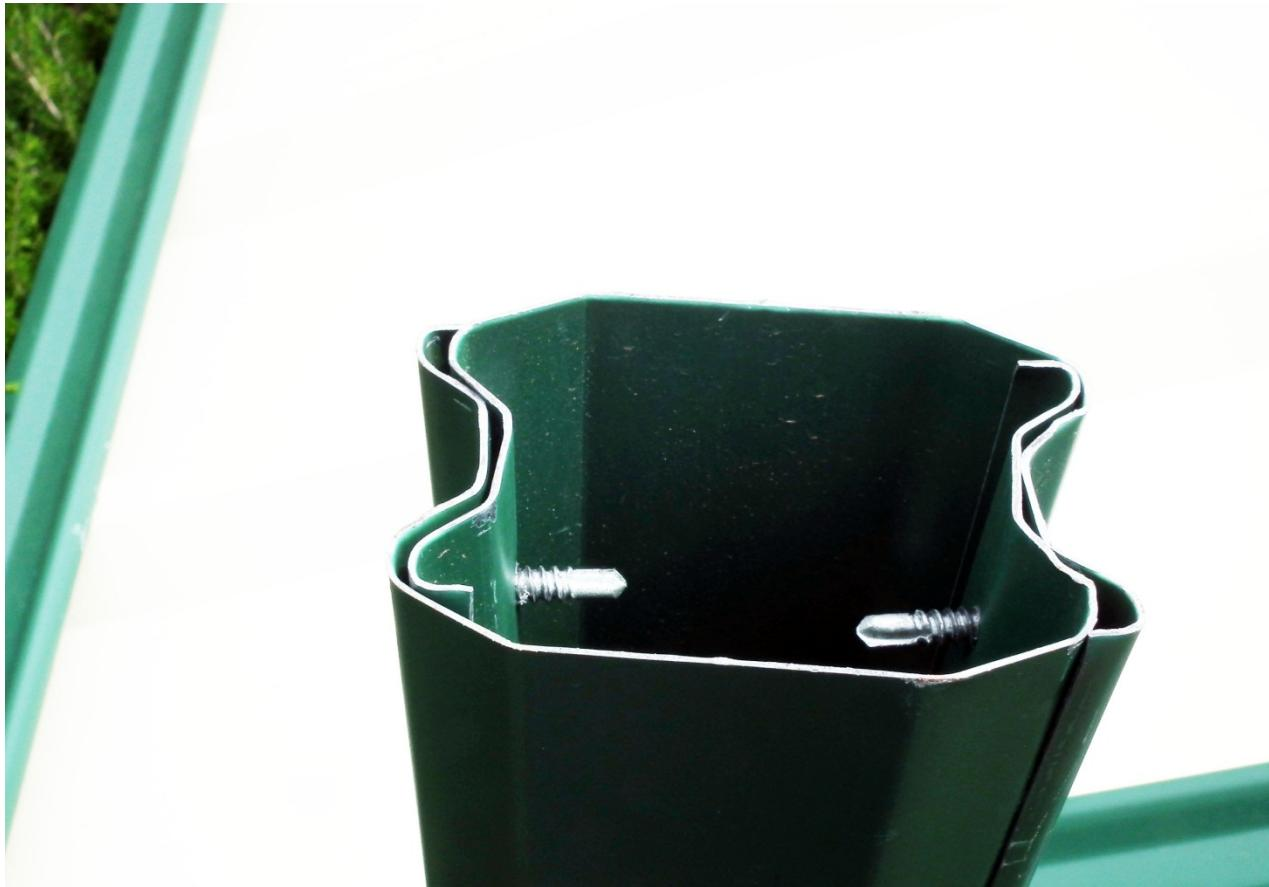
I left the sides their standard length, saves cutting them to size. Post has just had the “outer post” screwed in place as has the horizontal bracing.
