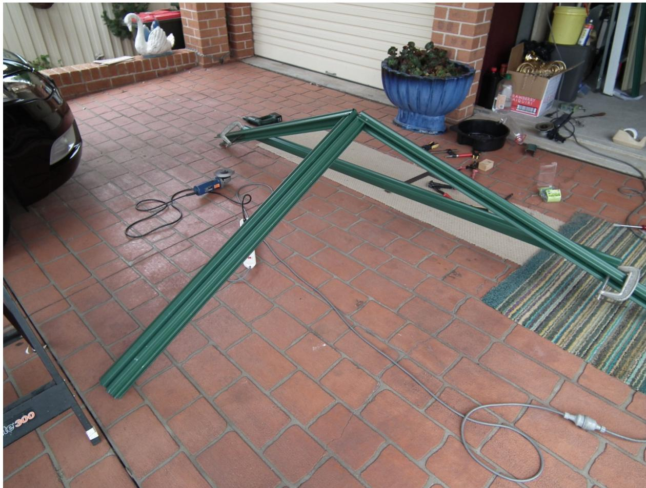
Two fence rails are riveted to form the roof ridge.
