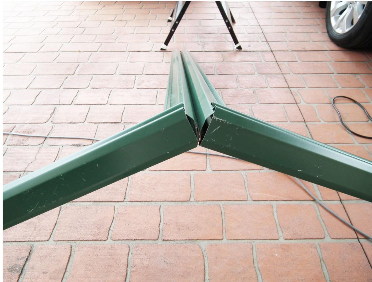
Close-up of roof rails pop riveted to fence posts, fence rails fit inside fence posts.
