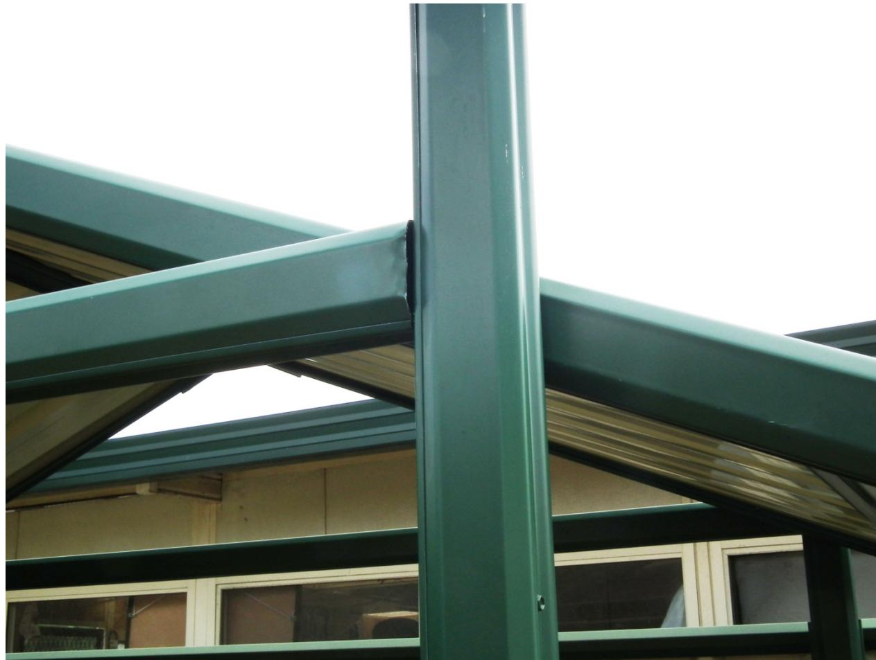
Two posts inside each other make a strong single post, The second post is only fitted after the first is already riveted to the "A" frame. Same applies to the two "A" frame bracing "rails", which are actually made from fence "posts".
