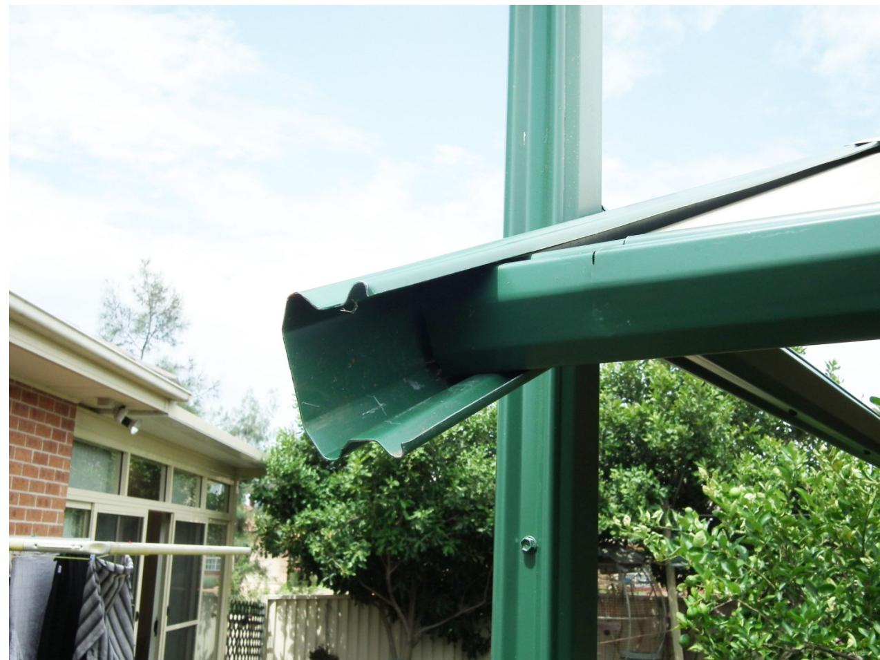
This view shows the bottom rail of the roof fitted in the side channels made from fencing “posts”. Four 3mm Galvanised steel pop rivets on top and bottom hold it all together.
