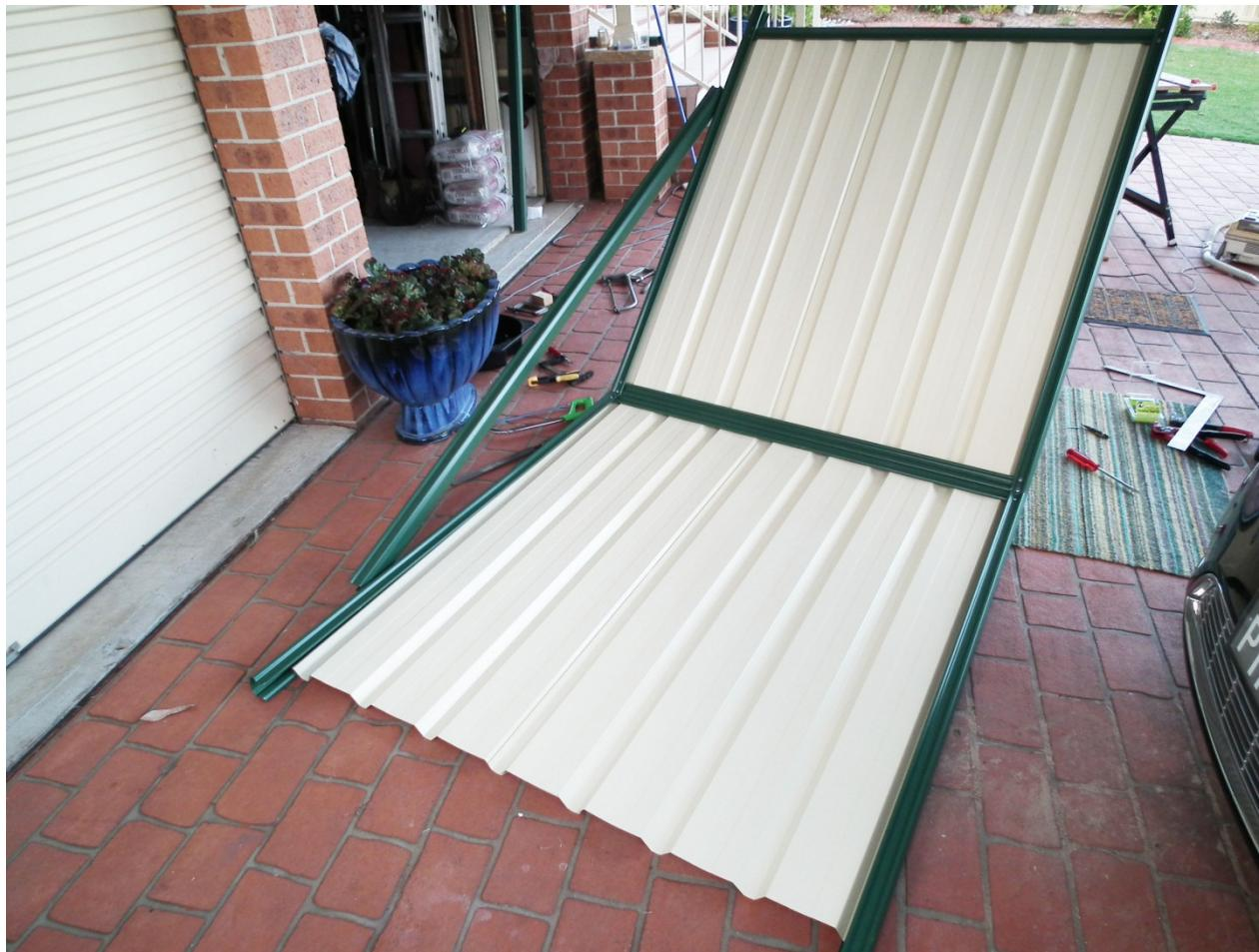
The finished roof with ridge cap folded over and pop riveted.
